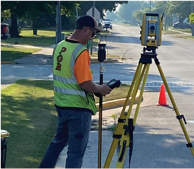
Point of Beginning Conducting Site Survey Work
