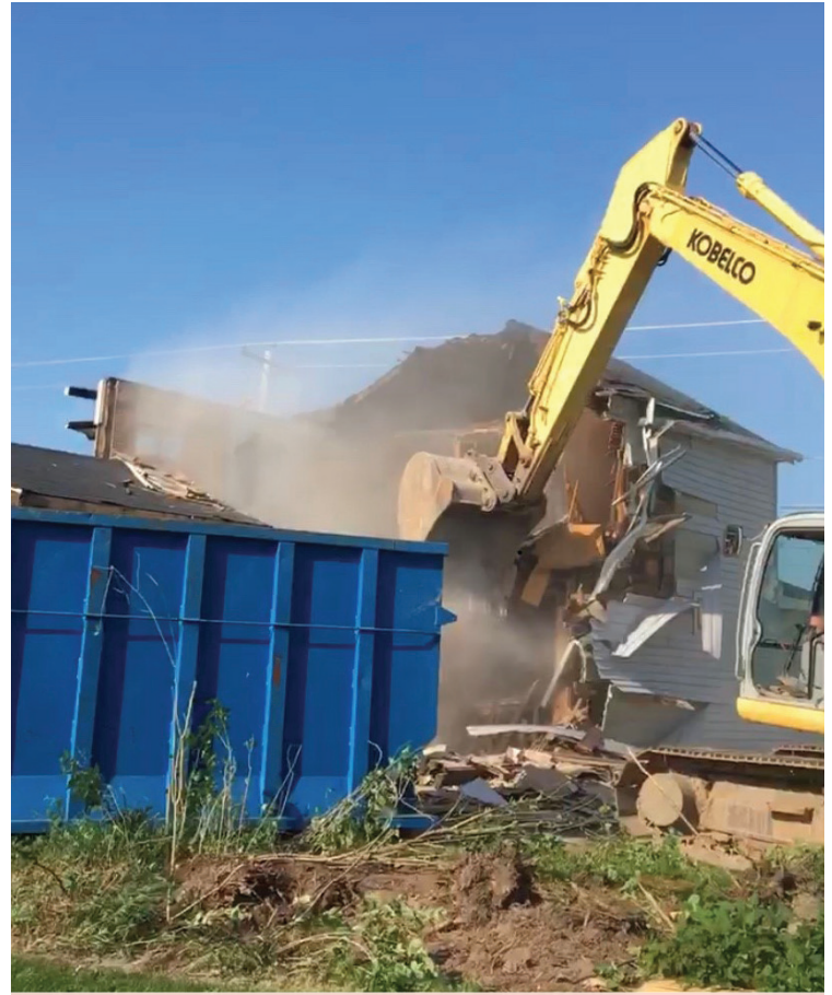
Demolishing the District-Purchased House on High Street
