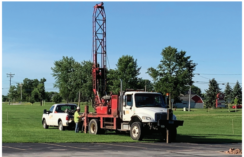
Soil Boring Work in Progress
