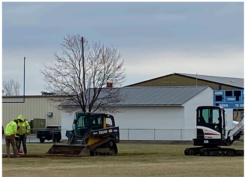
Replacement of Fiber Lines in Preparation for Construction
